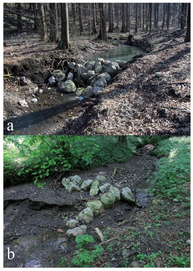
Fig. I Check dam at 1.7 river km of Libotínský potok – a) before the 5/2010 flood, b) after the 5/2010 flood
