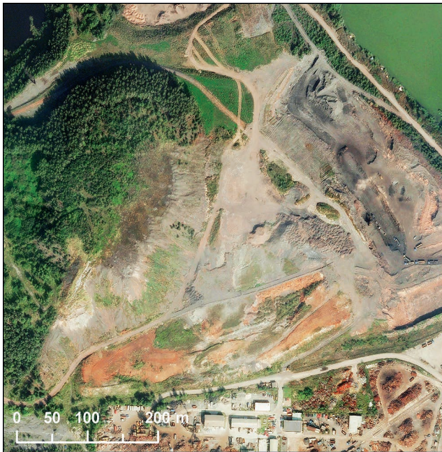
Fig. 18 Waste bank characterised by self-sustaining combustion in Heřmanice mining area (© GEODIS BRNO, spol. s r. o., 2009)
