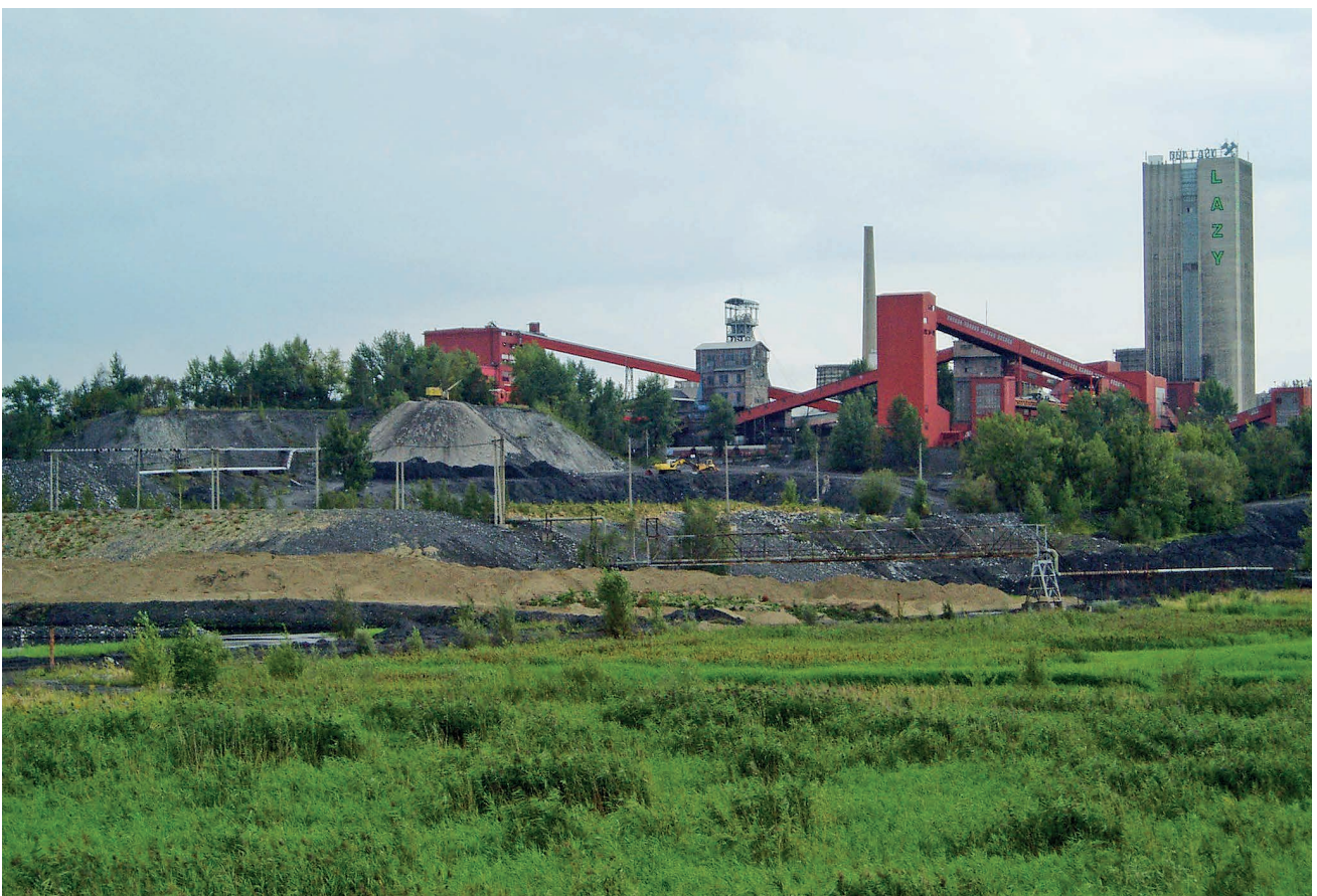
Fig. 23 Mine buildings of Lazy mine. Photo: M. Mulková, 2003
