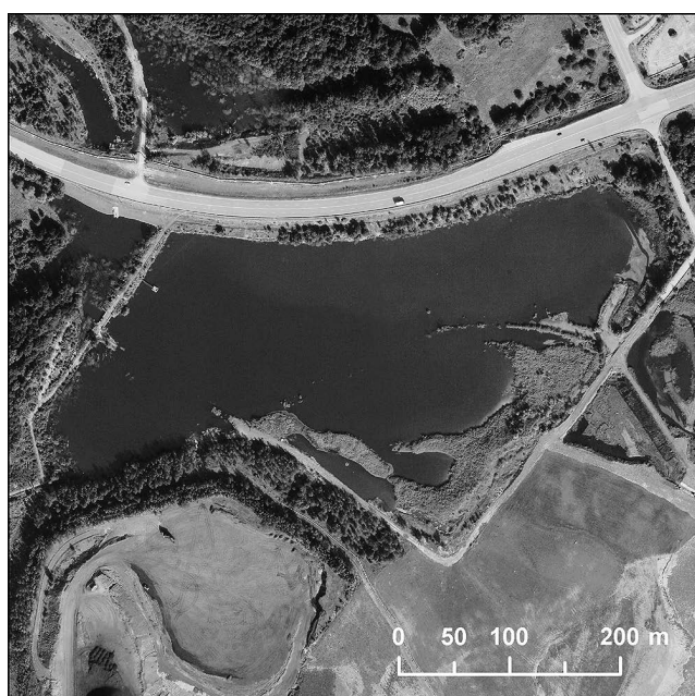
Fig. 6 Final sedimentation pond in Lazy mining area in an aerial photo from 2009 (© GEODIS BRNO, spol. s r. o.)
