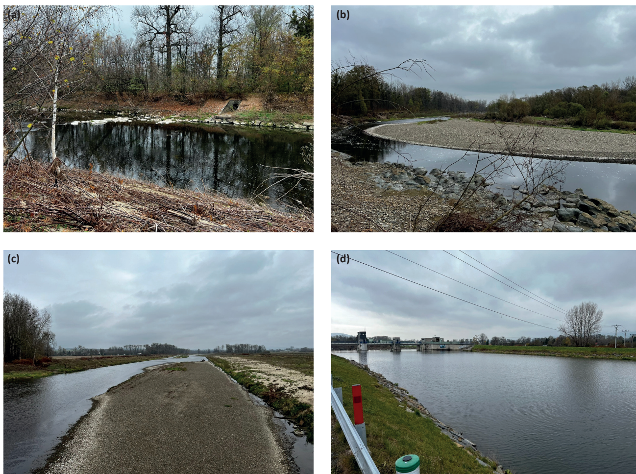
Fig. 2 Representative photographs illustrating the main morphological characteristics of the study reaches: (a) channelized reach CH1; (b) renaturalized reach RN1, developed following flood-induced embankment failures in 1997 and 2010; (c) recently restored reach RE; and (d) channelized reach CH5, strongly influenced by backwater effects associated with a weir.
