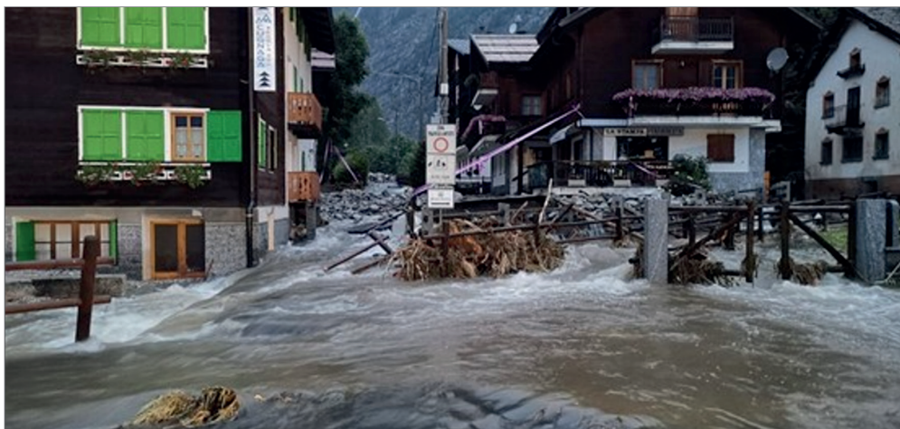
Fig. 2 Devastating flash flood from 2024 (Rio Tambach in the Staffa Village, part of Macugnaga), according Beba Schranz on www.nimbus.it .
