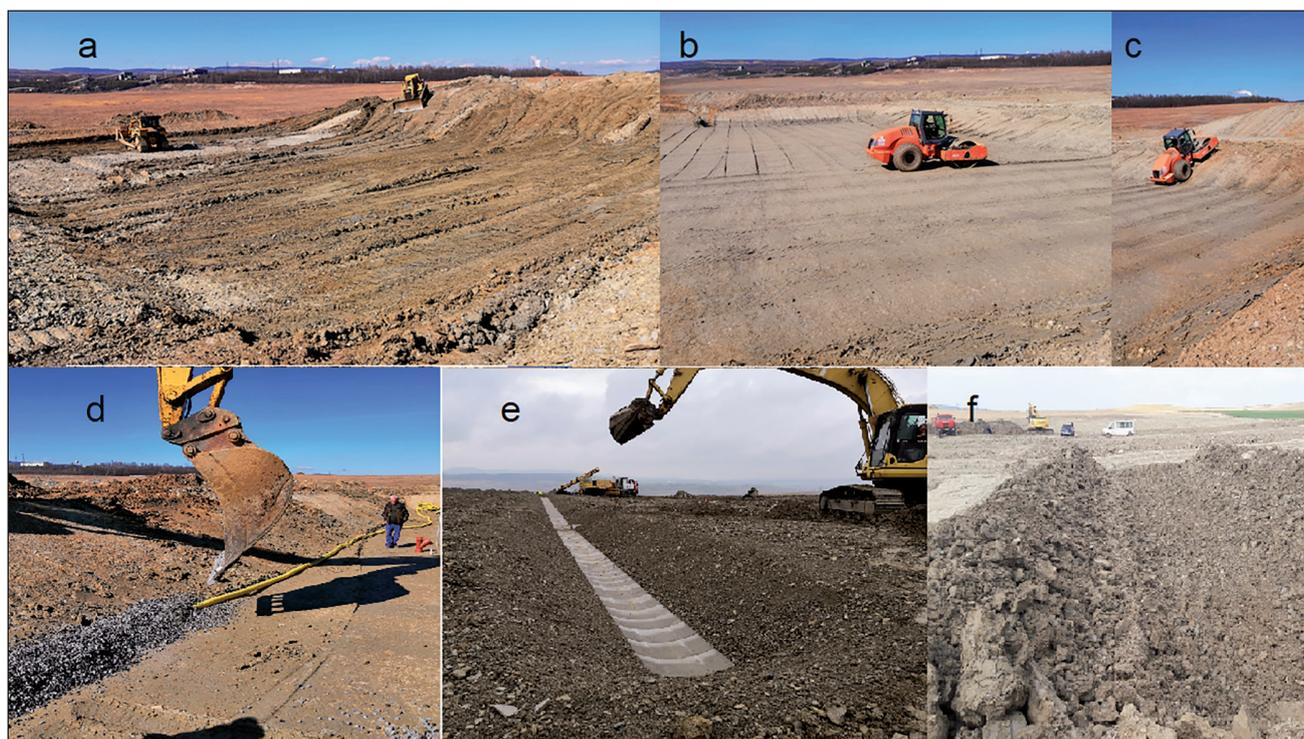
**Fig. 4** Key steps of catchment construction a) excavation, b,c) construction of sealing, d) construction of drainage system, e) detail of surface runoff collecting ditch, f) overall view on finished array.
